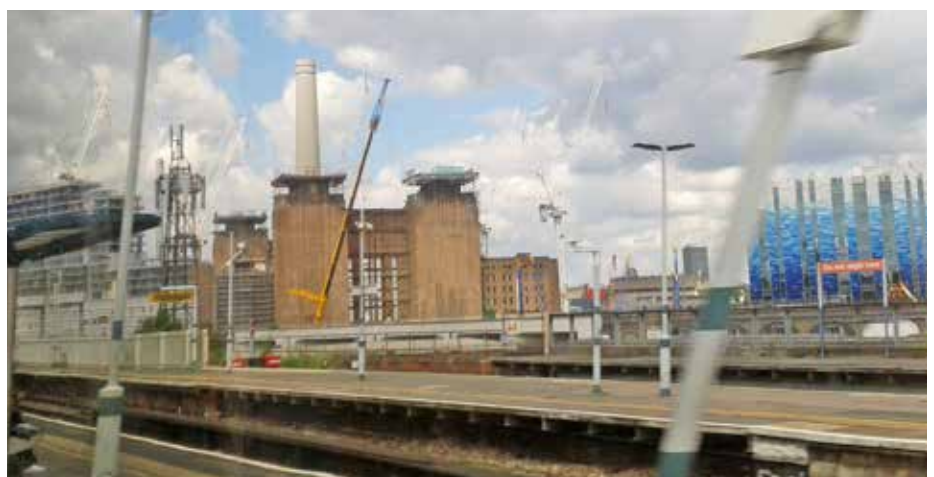
Umbau der Battersea Power Station (2016)
